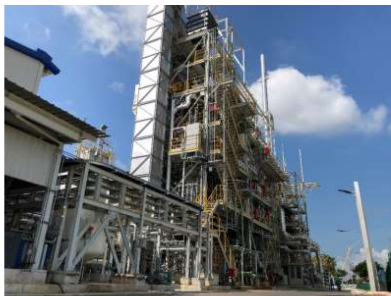
FE Shaft-Type Gasifying and Direct Melting Furnace (NTU-NEA WtE Research Facility)
