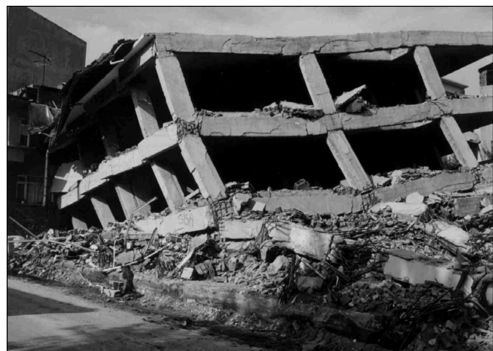
Severe damage to non-seismic detailed beam-column joints (Padang Earthquake, 2009)
